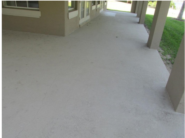
Patio floor surface with coating
