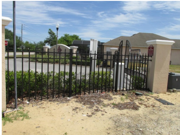
Fence at entrance
