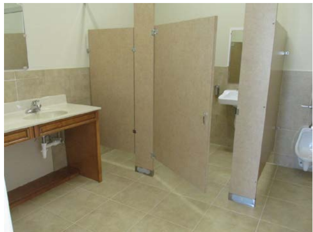
Rest room fixtures
