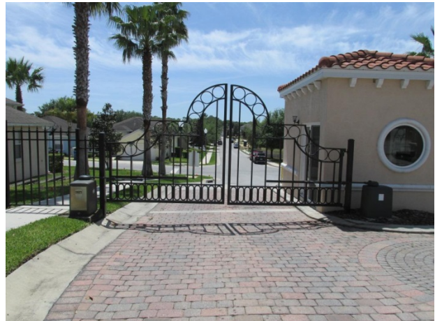
Main entrance gates and operators
