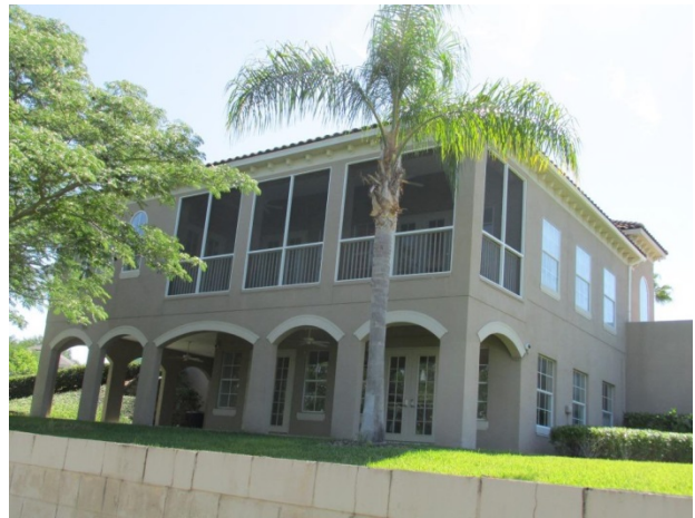
Rear elevation of clubhouse
