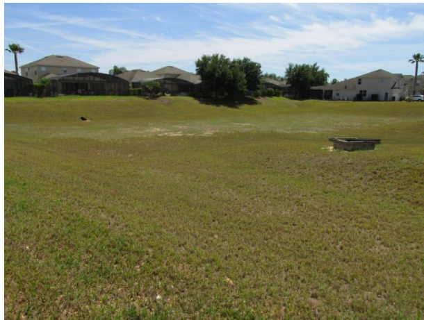
Overview of typical detention pond
