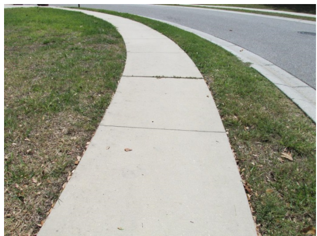
Typical concrete sidewalk
