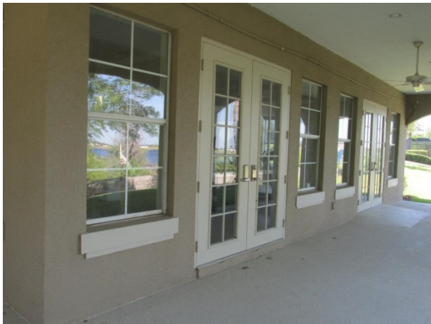
Windows and doors
