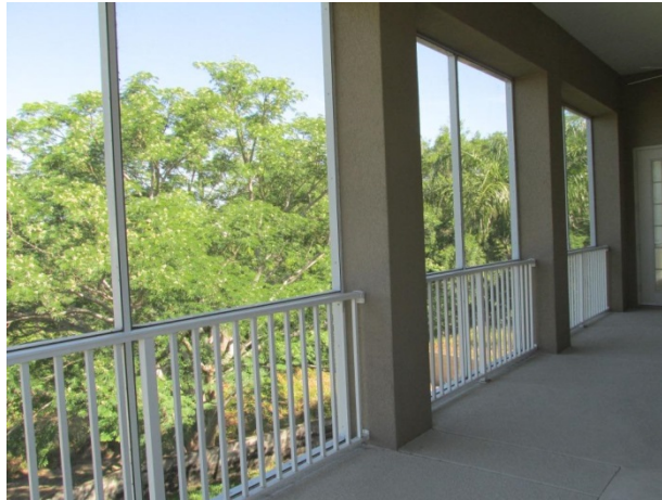
Balcony screen enclosure
